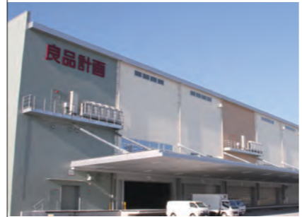
2014 Hatoyama Distribution Center
